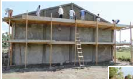
Nearing completion on shop-depot
